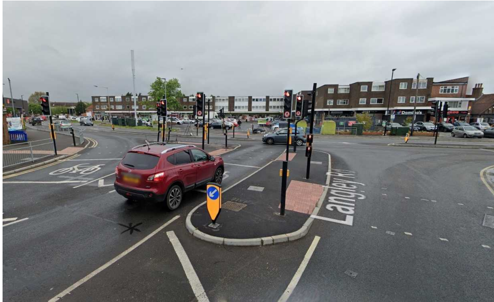
Approaching the new signalised junction at Harrow Market, from Langley Road
